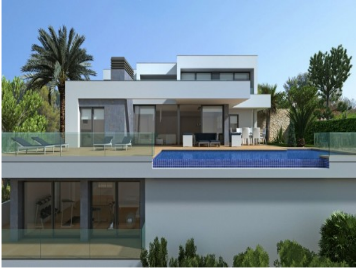
Front view of the villa with infinity pool
