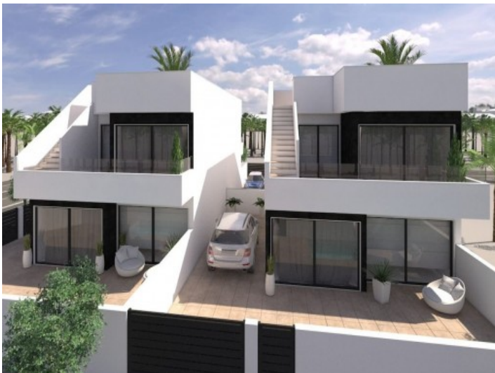
Parking lot next to the villa
